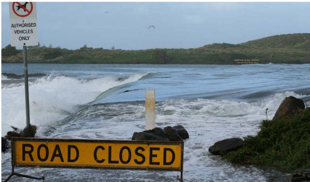
Figure 7: Differential wave setup over access road/breakwater/causeway to Griffiths Island May 2009 (James Phillips)
